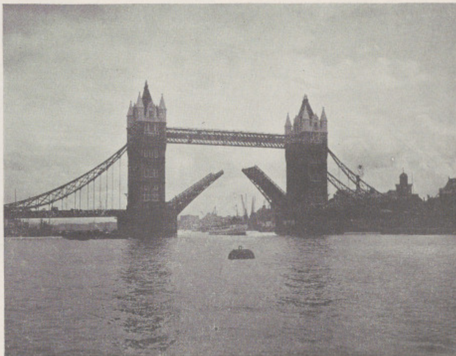
TOWER BRIDGE —Leading the Tower of London, the Tower Bridge is one of a series crossing the Thames, like the East River bridges in New York City.
